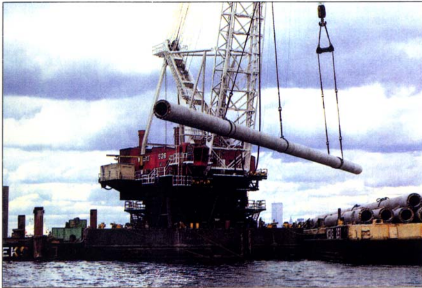
Left: Huge floating crane picks up piles believed to be the longest and heaviest cast to date. Right: Straight piles supersede battered piles.
