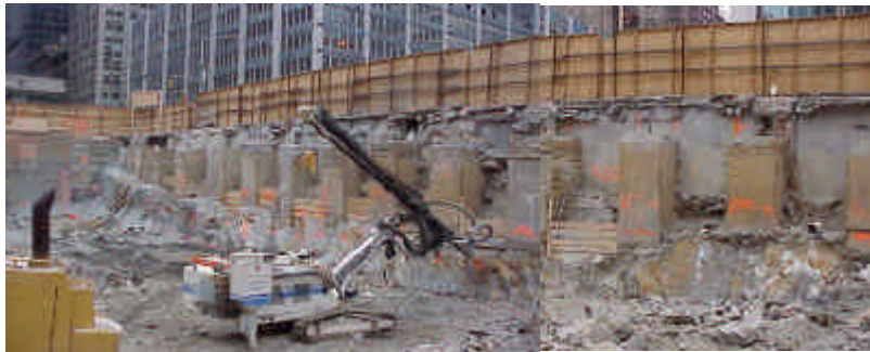
Top left: Rendering of the Bank of America Tower. Upper right plan shows location of the subways in relation to the site. Lower left: Excavation starting in October 2004. At corner of 6 th Avenue and 43 rd Street, rock anchors are drilled to support the subway which runs along 6 th Avenue. Lower right: At the bottom of the 60 ft. deep excavation in June 2005.
