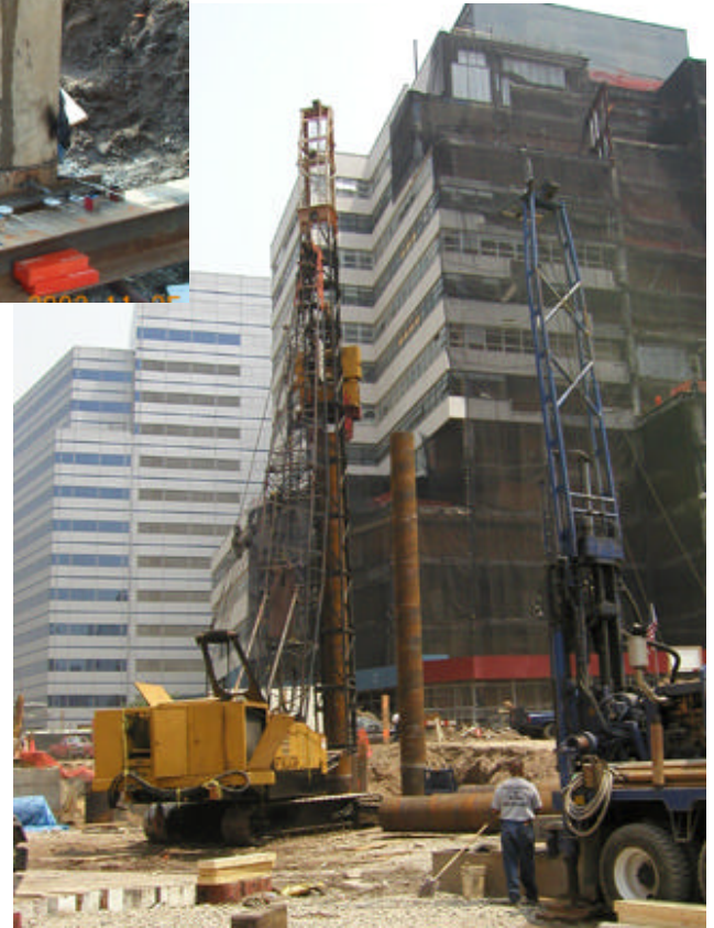
Clockwise from upper left: Model of new WTC; 50 ton max caisson lateral load test; installation of additional caissons from grade; general excavation and exposure of caissons.
