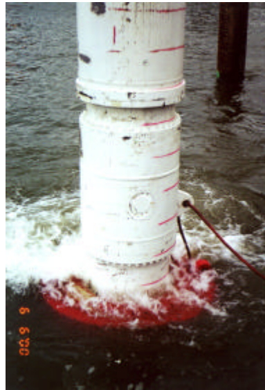
Top: Location of Bridge. Lower left: Potomac River Cofferdams. Center: Pile driving under water. Lower right: Production piles under construction and a static load test frame.
