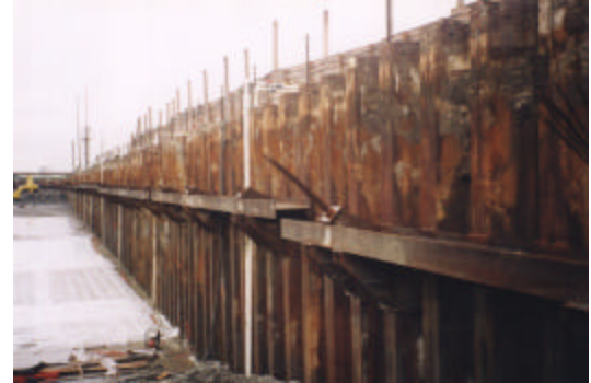
Above: Overhead view of the tunnel during construction. Above right: Sheet piling excavation support for the covered roadway tunnel. Lower right: Detail of wale and high capacity tieback system.
