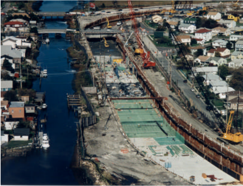
Above: Overhead view of the tunnel during construction. Above right: Sheet piling excavation support for the covered roadway tunnel. Lower right: Detail of wale and high capacity tieback system.
