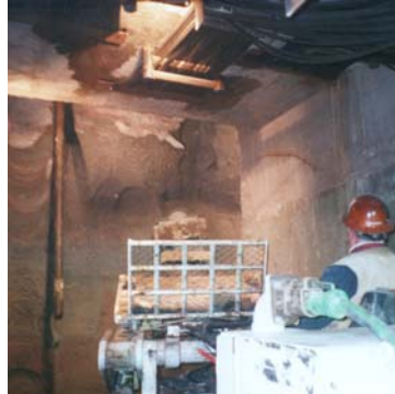
Left: Area where ground freezing occurred is pictured before construction began. Center: Frozen ground being excavated in the tunnel. Right: A 26m beam of frozen ground spanned the tunnel opening to prepare the cut-and-cover tunnel face for hole through of the last and longest jacked tunnel box. Insulated frozen ground supports the cut-and-cover excavation. The railroad above on the right is barely 6m from tunnel subgrade.
