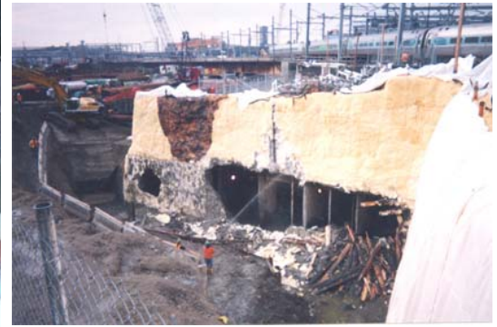
Left: Area where ground freezing occurred is pictured before construction began. Center: Frozen ground being excavated in the tunnel. Right: A 26m beam of frozen ground spanned the tunnel opening to prepare the cut-and-cover tunnel face for hole through of the last and longest jacked tunnel box. Insulated frozen ground supports the cut-and-cover excavation. The railroad above on the right is barely 6m from tunnel subgrade.
