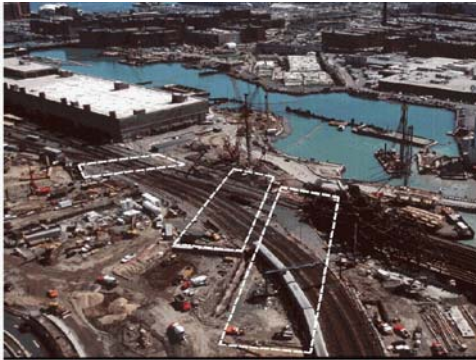
Left: Area where ground freezing occurred is pictured before construction began. Center: Frozen ground being excavated in the tunnel. Right: A 26m beam of frozen ground spanned the tunnel opening to prepare the cut-and-cover tunnel face for hole through of the last and longest jacked tunnel box. Insulated frozen ground supports the cut-and-cover excavation. The railroad above on the right is barely 6m from tunnel subgrade.
