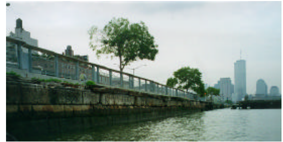
Lower Right: Bulkhead and platform structures at 45 th Street.
