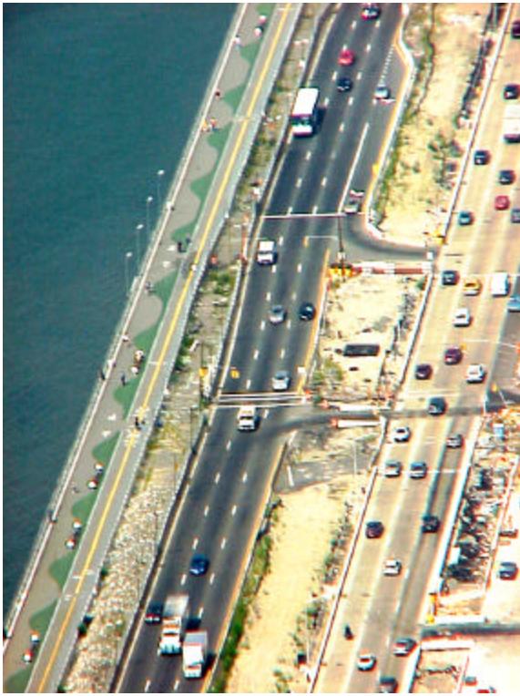
Left: Hudson River Park construction progressing in Fall 2000 along Route 9A.
