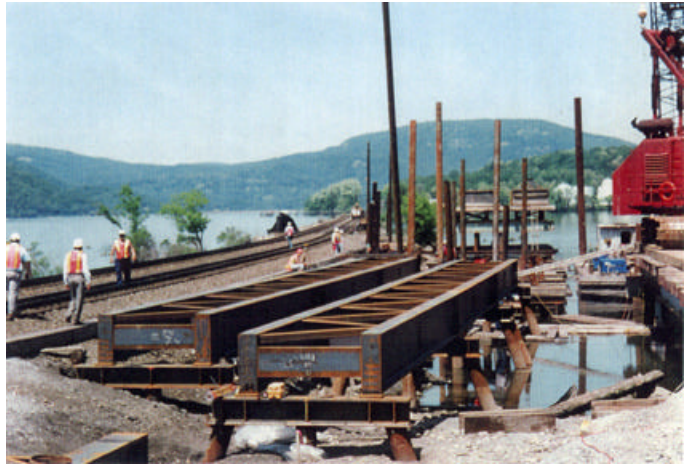
Construction of the temporary run-around trestle at Annsville Creek.
